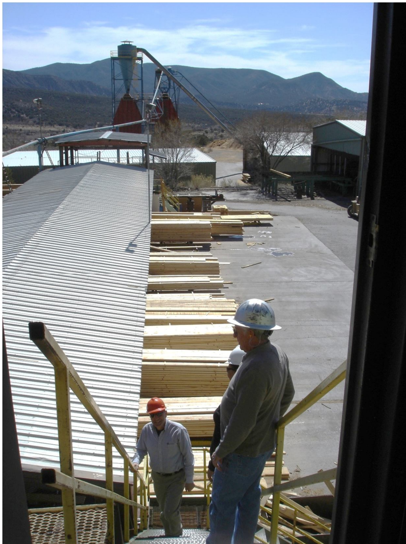
The green chain - Mescalero Apache. Photo by Larry Mason.
