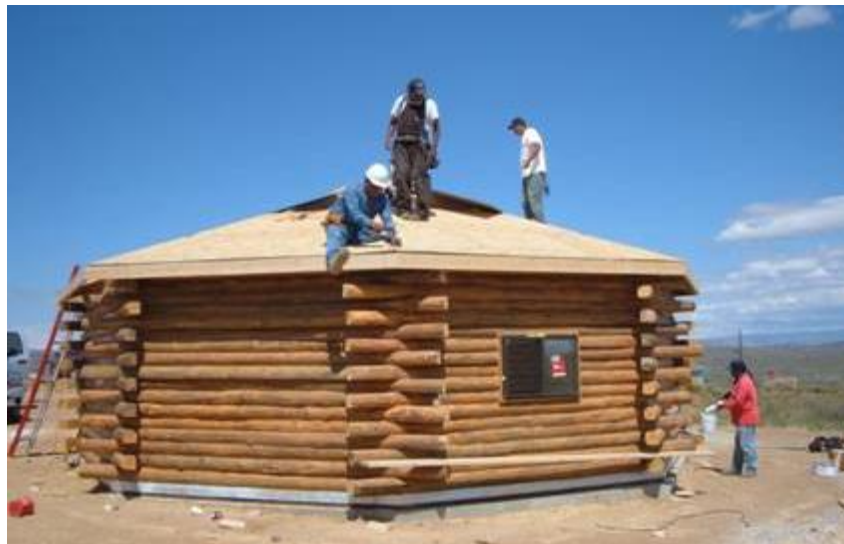
A Navajo traditional home, or hogan, being built with a Forest Service Collaborative Forest Restoration Program grant.
