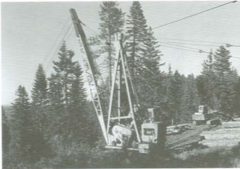
Cable logging. Yakima R.
