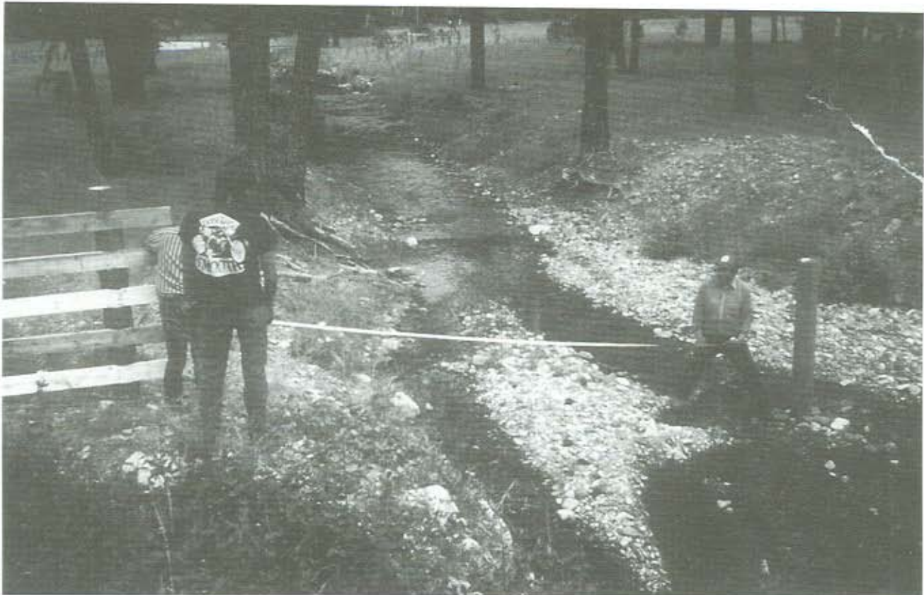
Stream restoration work. Colville Reservation
