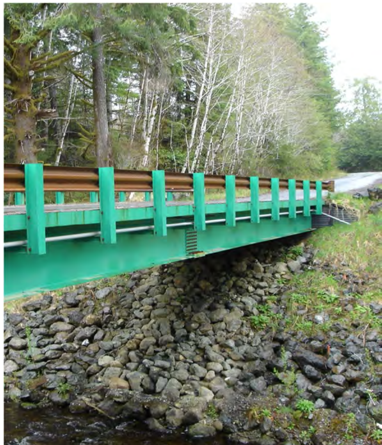
Bridge replacement funded with NRCS cost-share – Quinault. Photo by Larry Mason.
